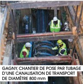
GAGNY, CHANTIER DE POSE PAR TUBAGE D'UNE CANALISATION DE TRANSPORT DE DIAMÈTRE 800 mm
